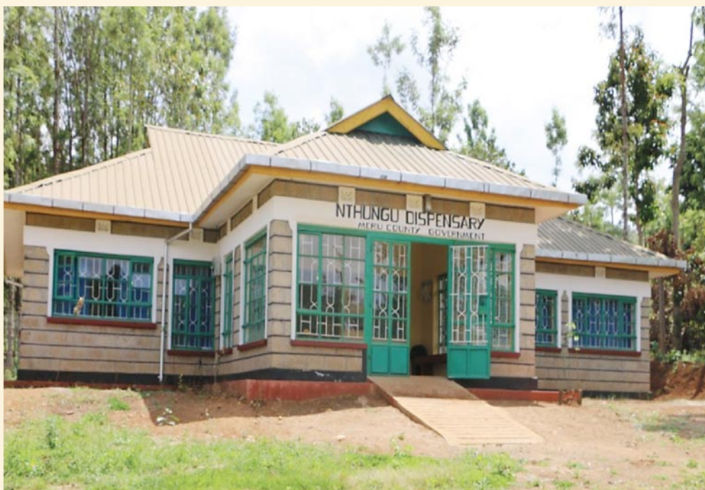
Nthungu Dispensary in Ntima West Ward, one of the many dis pensaries constructed by the County Government of Meru.
