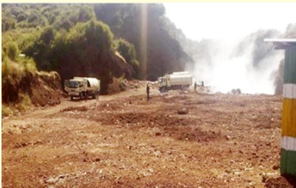
The rehabilitated Nkunga dumpsite.
