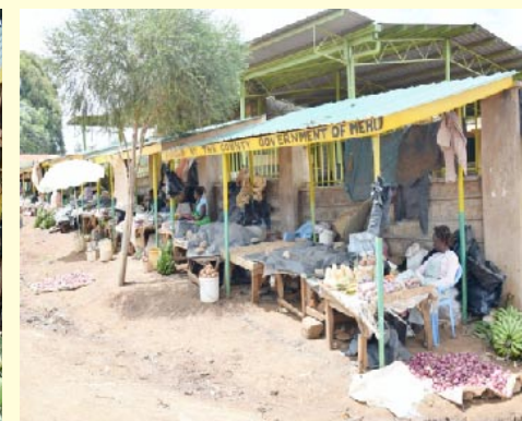
One of many market sheds constructed by County Government of Meru.
