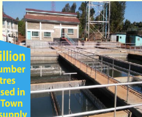
Water treatment plant at Meru.
