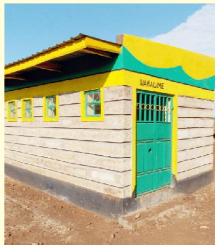
One of many public toilets constructed.
