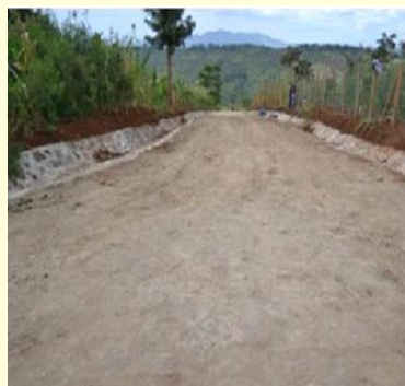
Improved access road to Muungu dumpsite.
