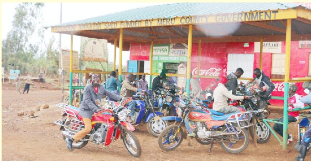
Boda Boda shed constructed by the County Government.
