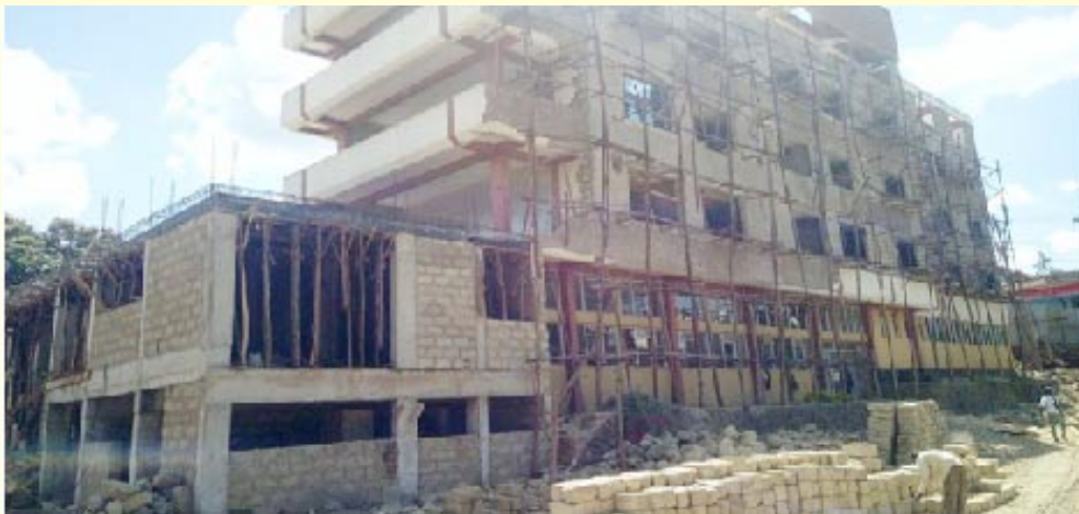
The ongoing refurbishment works at Meru County Hotel to convert it to an ultra-modern three-star hotel.
