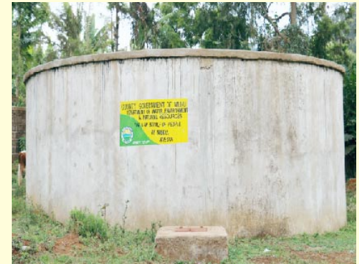
Water tank constructed at Kiegoi area.
