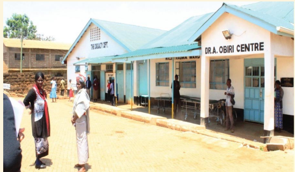
Cabro paving of the Hospital parking at MT&RH.
